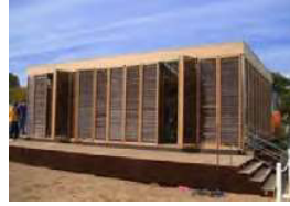
Kinetic shutters allow for shade in summer and solar gain in winter
